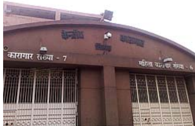
Bosch AutoDome camera installed at one of the Prisons of Tihar Jail..
